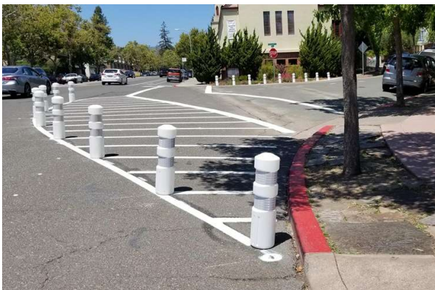
Crossing improvements at Grand Avenue/Fairview Avenue.
