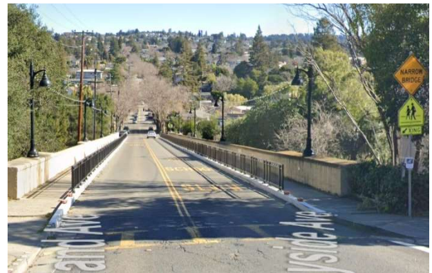
Sidewalk railings on the Oakland Avenue bridge.
