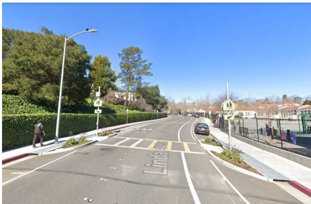
Bulbouts on Linda Avenue along Linda Playground.
